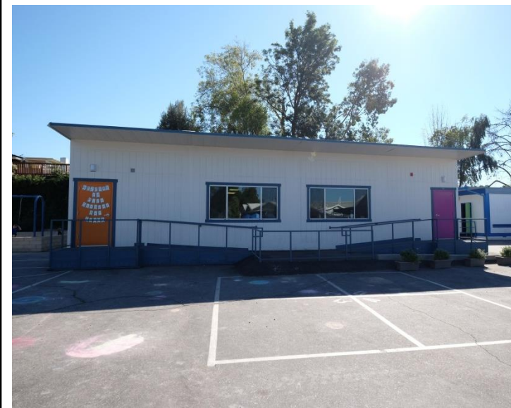
Photo 23 Building Name: Classrooms (Modular) Building Number: 8 Built 2016, Classroom and Science room
