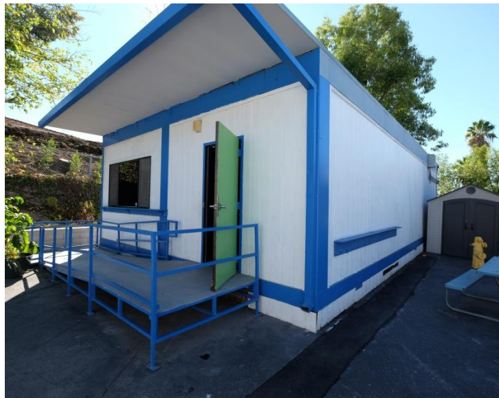
Photo 21 Building Name: Classroom (Modular) Building Number: 7 Music
