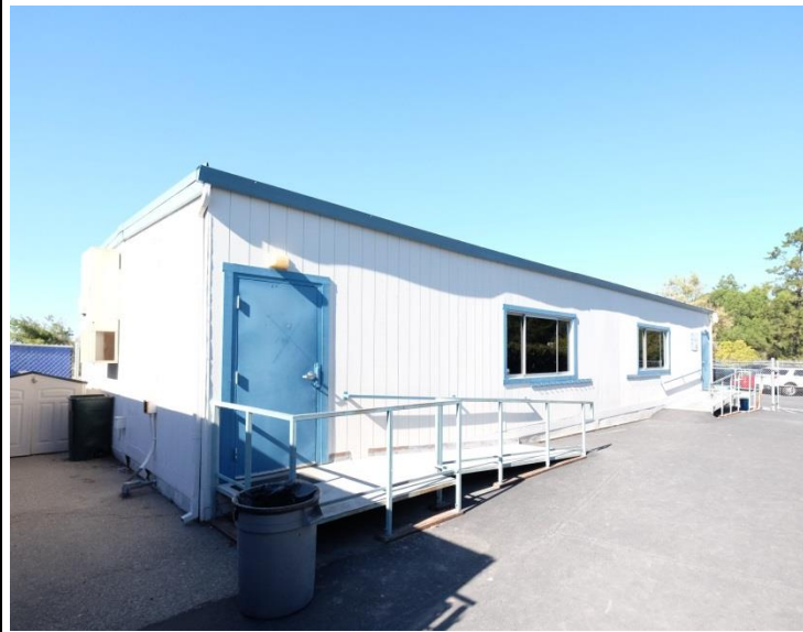
Photo 9 Building Name: Child Care Building Number: 2 Exterior view of portable building
