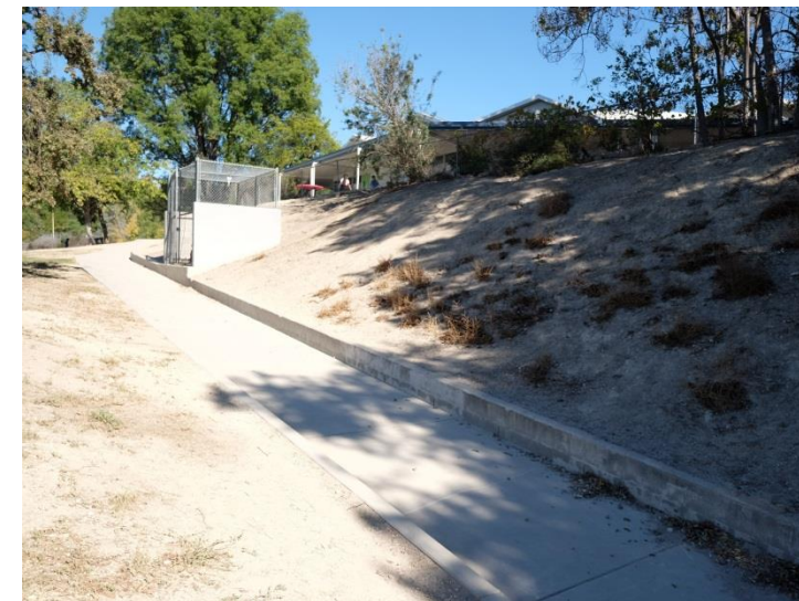
Photo -5 Walkway from back entrance up to campus. Not a ADA accessible path.
