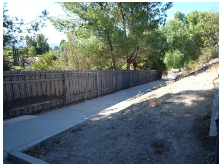
Photo -3 Walkway from back entrance off of Falmouth St. up to campus. Not an ADA accessible path.
