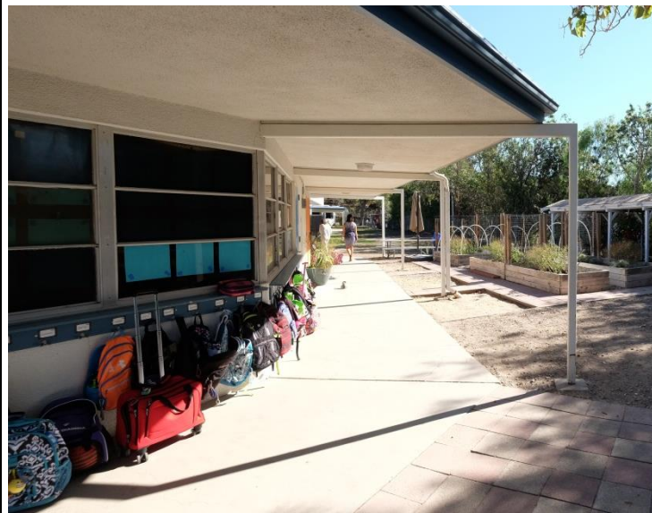
Photo 13 Building Name: Classrooms Building Number: 4 Building 4 and adjacent garden
