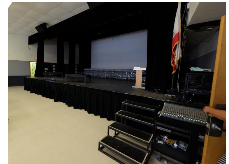
Photo -6 No wheelchair lift provided to stage.
