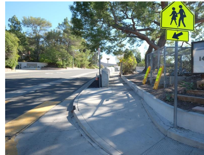
Photo -1 Main drop-off on La Granada Drive. Children walk along the left side of the wall when dropped off at the curb. Walkway is too narrow and not safe.
